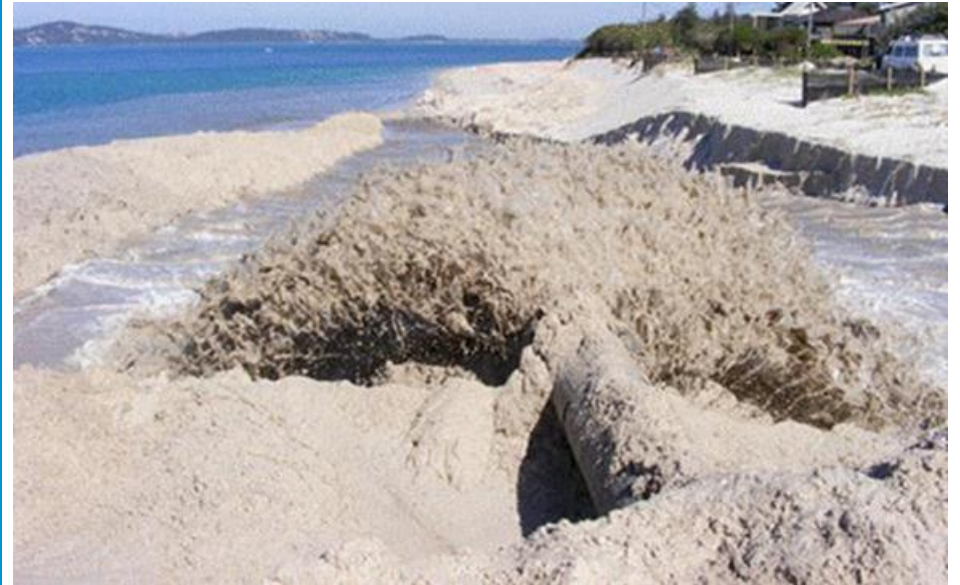
Figure 26: Beach renourishment has been combined with revegetation to manage coastal erosion, in this case at Jimmys Beach, Port Stephens
