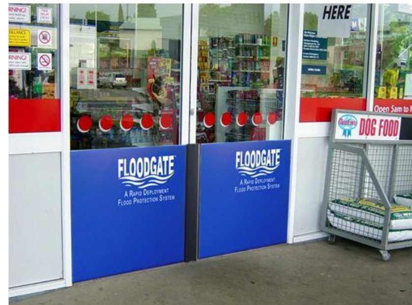
Flood barrier, Swansea Caltex
