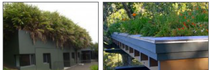
Figure 6: Green roofs in a commercial and urban setting
