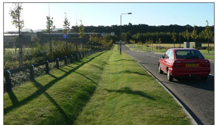
Figure 8: Roadside swale. (Source: Dr Scott Arthur).
