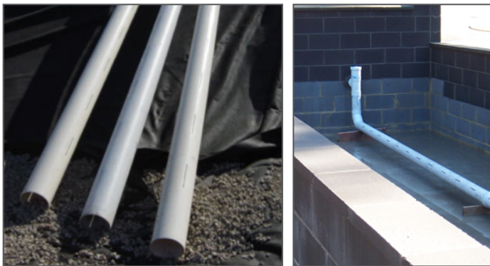
Slotted pipe used for subsurface drainage
