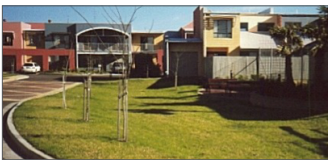
Urban detention and infiltration basin under normal conditions.
