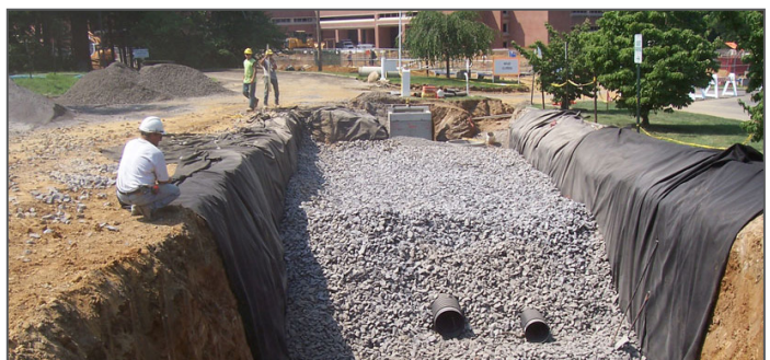
Figure 10: Large infiltration trench construction. (Source: Temple Villanove Sustainable Stormwater Initiative).
