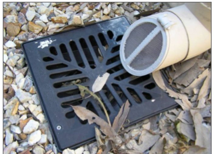
Mesh screen over the tank overflow pipe
