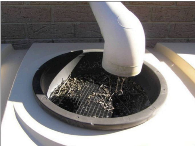
Figure 11: Clean inlet screen in tank (Photo courtesy of Lake Macquarie City Council)
