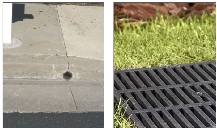
Figure 7: House drainage can be connected to either the the street and kerb (left) or the rear of the property (right).
