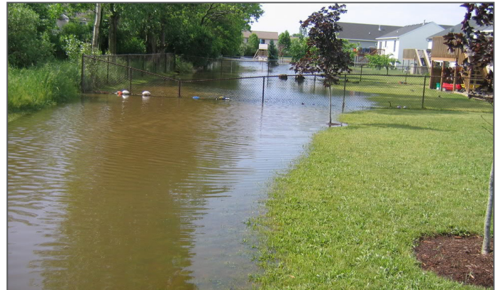
Figure 6: In some situations, floodways and overland flow paths are required around the home. (Source: Lanai beach blogspot).
